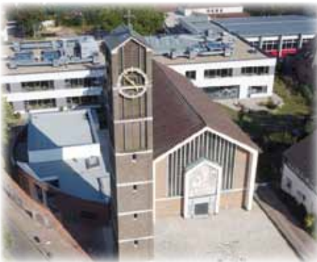
(Foto: Marc Wattering)
